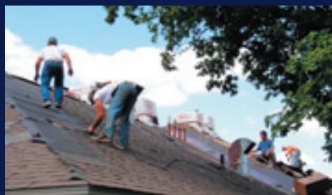
Re-roofing the Stans Museum
